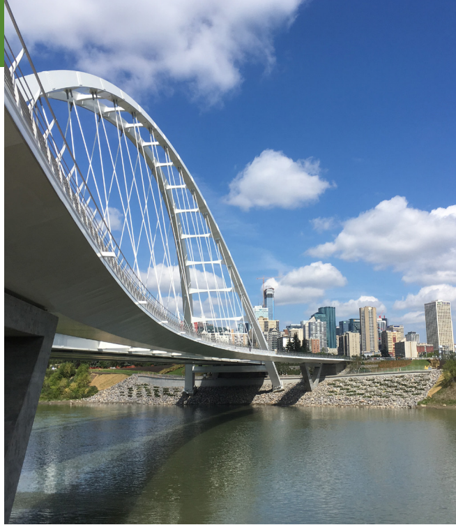
WALTERDALE BRIDGE REPLACEMENT, EDMONTON, AB
