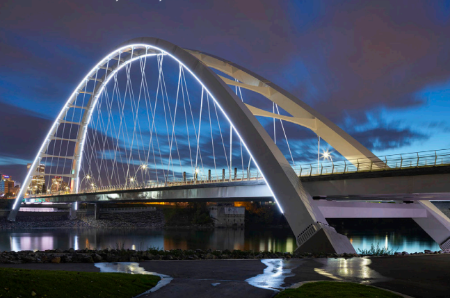
WALTERDALE BRIDGE REPLACEMENT, EDMONTON, AB
