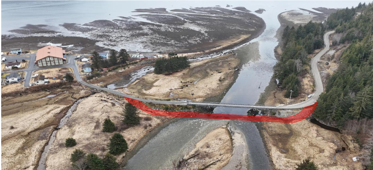
Figure 2: Aerial view looking south showing the approximate upstream alignment of the new bridge highlighted in red, relative to the existing Ksi Gingolx Bridge and surrounding site features.
