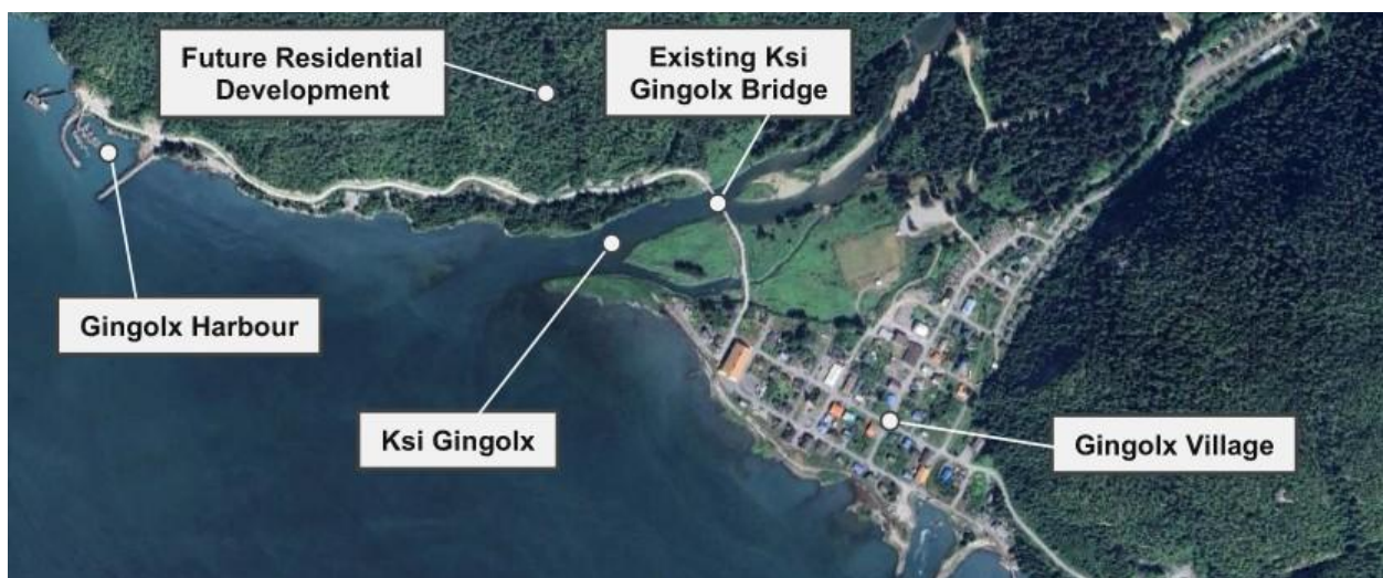
Figure 1: Aerial view of the Village of Gingolx showing the Ksi Gingolx River, the existing bridge crossing, Gingolx Harbour, and surrounding development areas referenced in the project scope.
