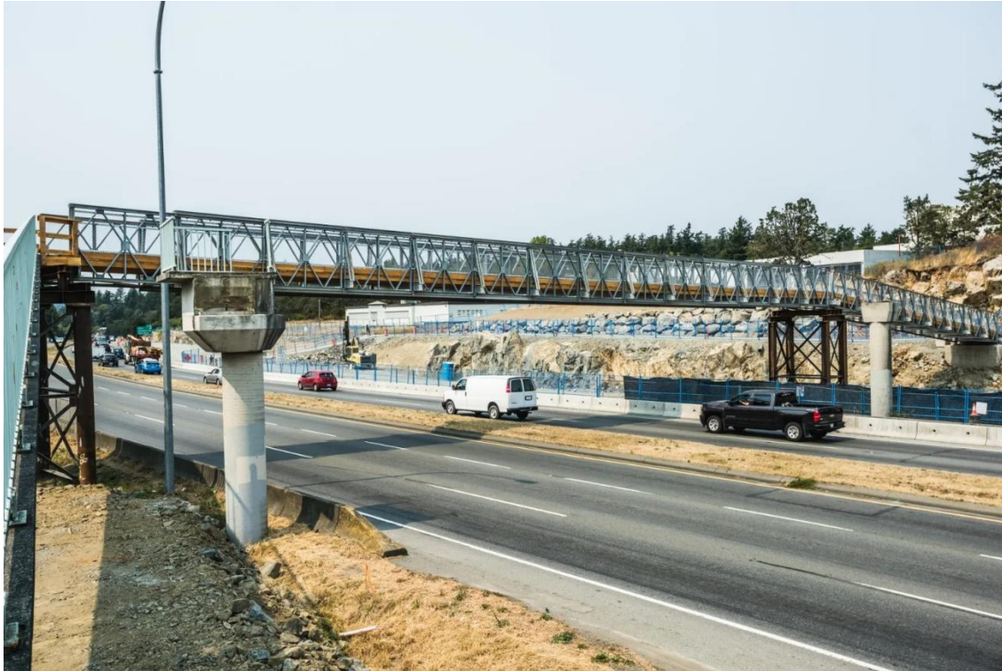
Figure 4: MABEY C200 truss segments in their previous deployment at the Admirals-McKenzie Interchange Project, prior to acquisition for reuse at the Tsolum River Bridge (BC MoTT, Jacob Bros Construction).
