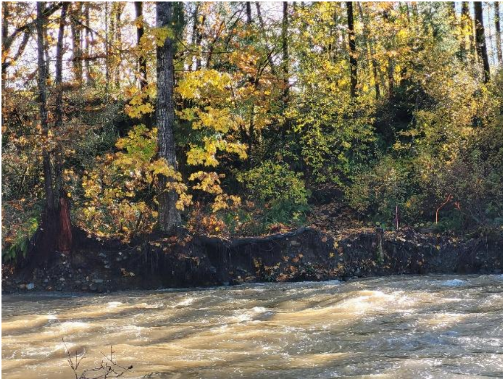
Figure 3: Ground-level view of the Tsolum River during a 2026 flood event.
