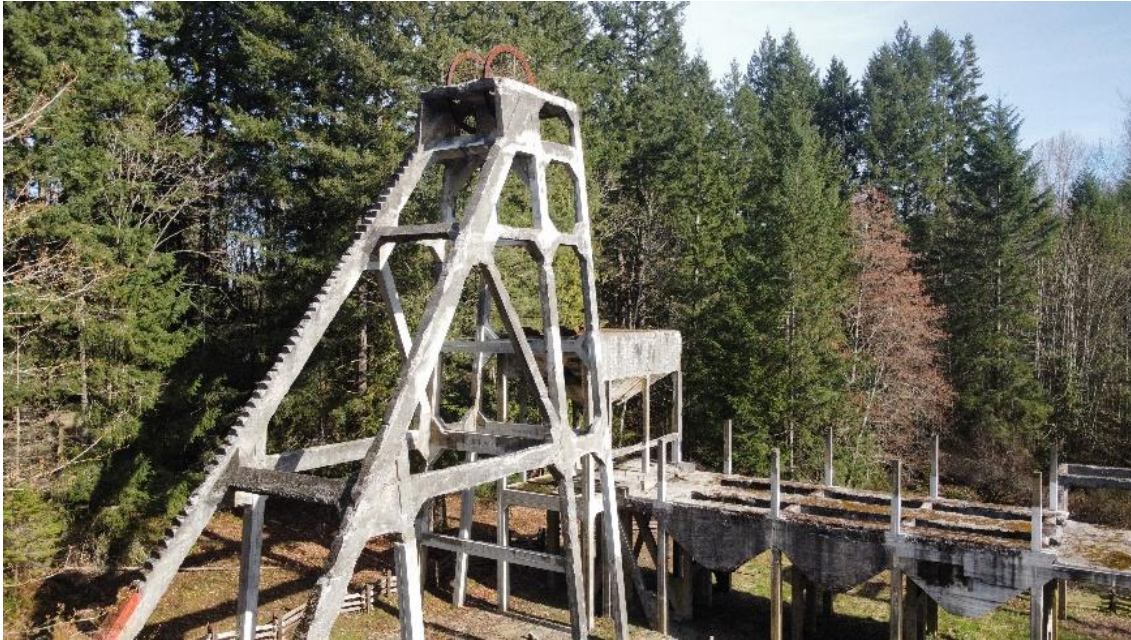
Figure 7: The Morden Colliery reinforced concrete headframe and tippie, showing the iron wheel at the crown of the headframe.
