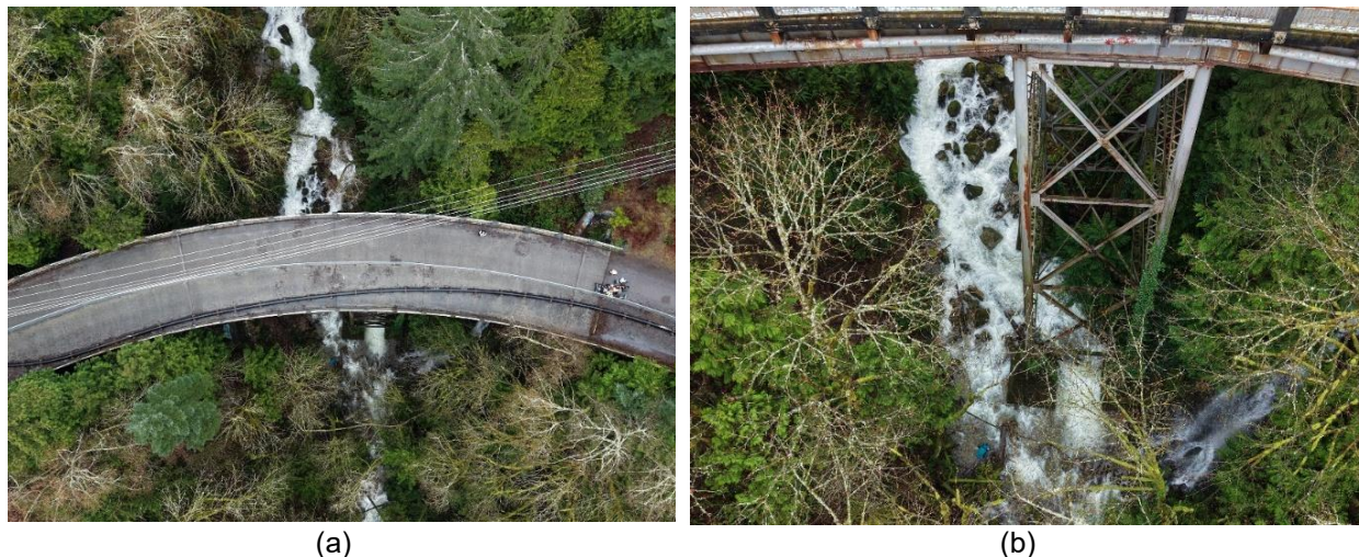
Figure 1: Nelson Canyon Bridge (Existing Structure) a) top view - superstructure b) steel truss pier substructure
