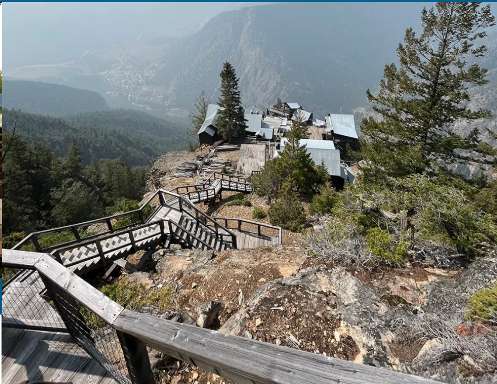
BRAZEAU COLLIERIES STRUCTURAL PRESERVATION, NORDEGG, AB
